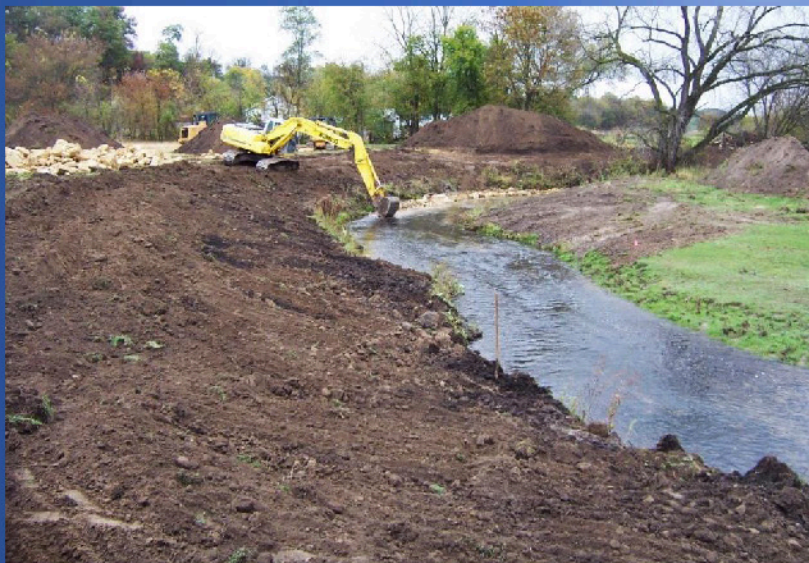
Streambank Stabilization
