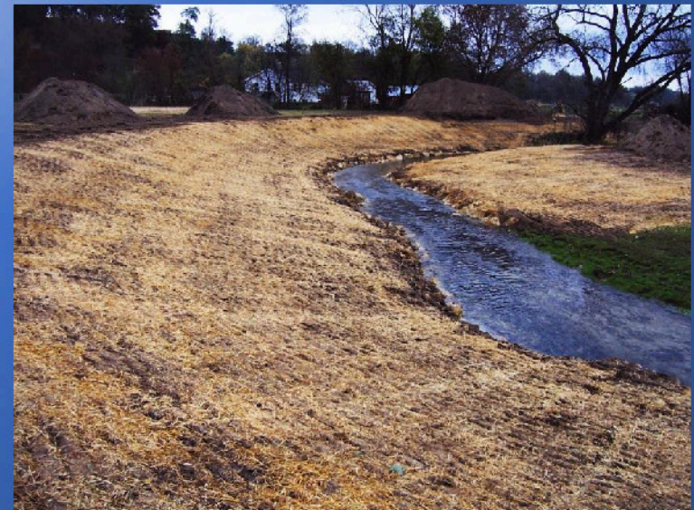
Streambank Stabilization
